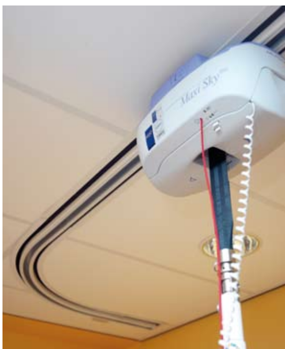
The track can be partially concealed in a suspended ceiling to provide a discreet solution.
